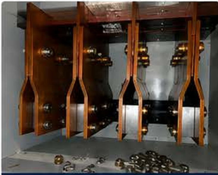
EXISTING LV BUSBAR WORKS
