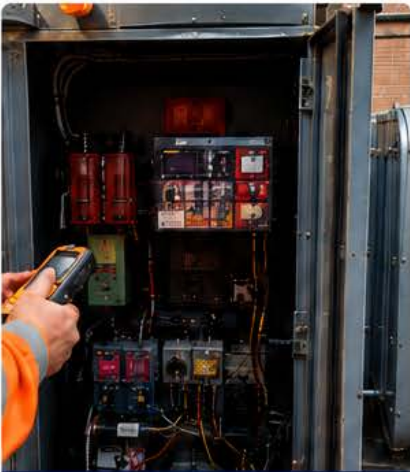
PROTECTION TESTING & COMMISSIONING
