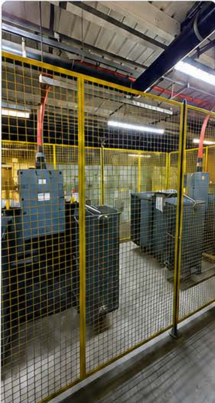
TRANSFORMER B – OIL REPLACEMENT & MAINTENANCE WORKS
